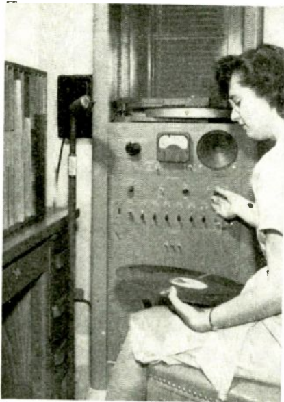
Amplifier and control rack in anteroom distribute music through Stouffer's, Cleveland.
