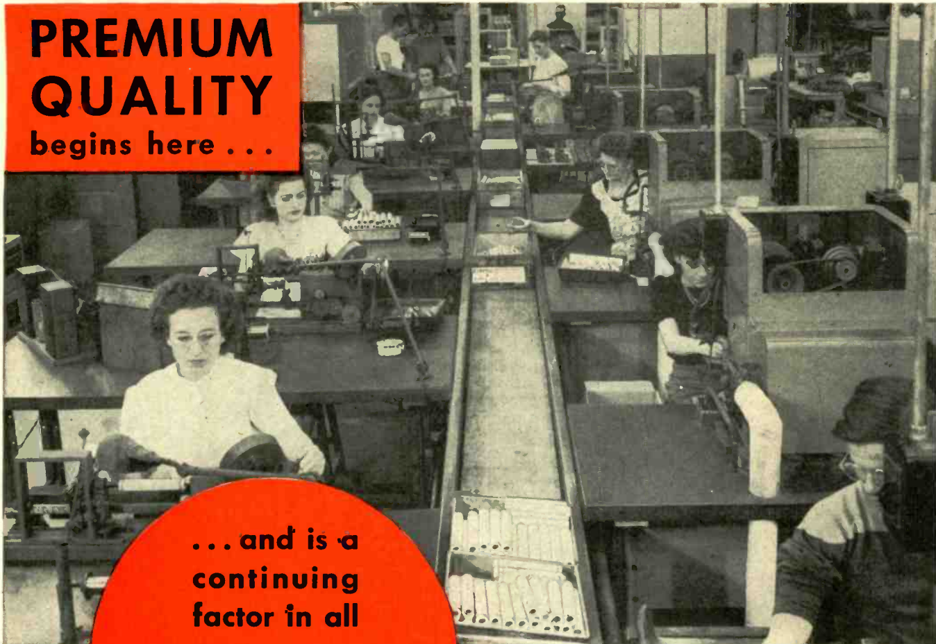
(Above) Mallory operators wind resistance wire on vitreous enamel resistors. This is a precision job. Operators chalk numbers of turns being wound by use of gauge. Resistance value of each resistor is kept within rigid tolerance specifications. Note the straight line production set up. After resistors are wound and welded, they move on to enameling and baking operations in the background.
