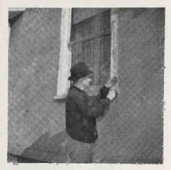
Check antenna and lead-in connections.
