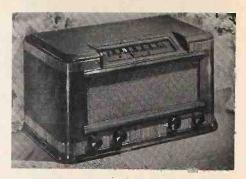
inet and provide correct voltages. Automatic volume control,  $6^{1}/2^{\prime\prime}$  PM speaker driven by beam-power amplifier. Slide rule dial with large numerals. Walnut veneer cabinet with oriental walnut banding and harmonizing center panel of grille cloth. \$38.80 in Zone 1. The Hallicrafters Co., 2611 S. Indiana Ave., Chicago, Ill.—RADIO & Television RETAILING
