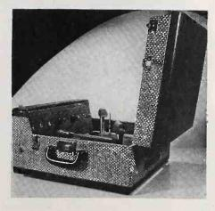
Model MC-2 automatic record player, portable type. Three tubes, ac. De luxe 2-post automatic changer, Alnico 5 speaker. Controls on tilted panel. Televox, Inc., 451 S. 5th Ave., Mt. Vernon, N. Y.—RADIO & Television RETAILING
