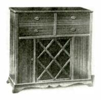
Model 22-APR, automatic radio phonograph console combination, ac superhet with both broadcast and short wave bands. Push-pull beam power output, built-in loop antenna, variable tone control, 7 tubes including rectifier. Mahogany cabinet with slide drawer record changer compartment and record storage space. Telicon Corp., 851 Madison Ave., New York 21, N. Y.--RADIO & Television RETAILING
