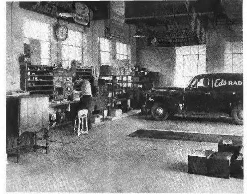
Here again, Ed has allowed plenty of space for enlargement. This up-to-the-minute, fire-proof garage has room enough for four cars and a special radio repair bench for auto radio work, as well as metal rack stock space for parts.
