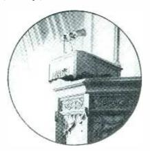
SPEAKER—One horn (right) does entire job, is mounted in decorative housing suspended 20 feet from floor in center of Gothic arch above the pulpin
