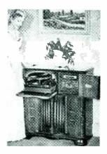
RCA CONSOLE COMBINATION RADIO with automatic "Magic Brain" victrola, model V-215, has 9-tube radio, 3-band chassis. 12-watts output. Record changer rolls out of the cabinet when the phonograph compartment is opened. Mechanism is completely automatic, no need to touch the tone arm or shut the mechanism off. Cabinet is built of matched walnut and managany veneers. RCA Mfg. Co., Camden, N. J.
