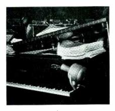
PIANO—In the Grille of the Hotel New Yorker, a tiny contact pickup is mounted inside the piano. That knob, just above the keyboard, adjusts volume source in order to avoid feedback.
