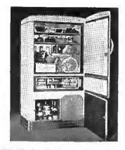
STEWART-WARNER 871 Pural Temp, deluxe, ator is equipped with a freezing locker to-cated near the center of the refrigerator with 5 snapout Ice trays (one of double width); 4 shelves including 2 sliding shelves and 4 removable sections; vegetable basket; dry storage cabinet. Price \$259,75. Stewart-Warner Corp., Chicago, III.
