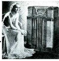
MODEL BC-102—A 10-tube superhet with 3 wave bands tuning from 540 kc. to 18.1 mc. Contains shielded rotable Built-In-Tenna; automatic volume control; bass compensation; 12 inch dynamic speaker; 10 watts output; provision for television and phono. Cabinet finished in American stump walnut with rare wood inlays.
