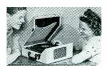
PHONOGRAPH AND RECORD PLAYER — Completely self contained, fully portable electric phonograph is also a remote operating wireless record player suitable for use with any radio. Has crystal pickup, self starting constant speed motor, permanent magnet dynamic speaker, cloth covered portable case.
