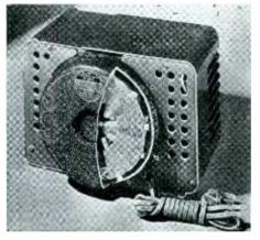
AEROSCOPE—Low-loss spiderweb winding method makes for good signal pickup as well as compactness in Admiral's 161-5L.
