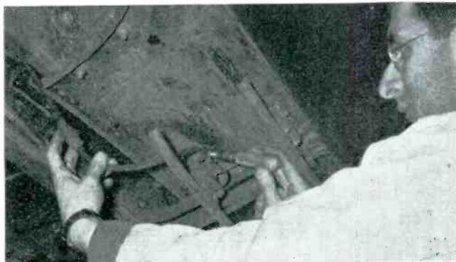
GROUND SHIELDING —Short ground leads essential on undercar systems. Shield connection (center) grounds on running-board two inches from antenna. Taped connection (left) grounds shield to car frame.
