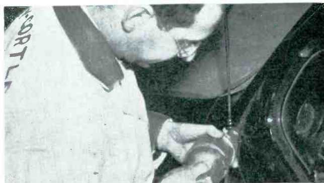
WHIP NECESSITY —With door slightly ajar drill hole in body channel to lead in whip-type antenna; otherwise channel construction cuts wire insulation.
