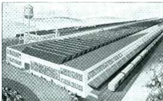
Shown above is the recently completed first unit of four to be built by Crosley on the 90-acre tract at Richmond, Ind. This first unit, 200 feet wide by 1200 feet long, is the last word in production efficiency with a capacity of 1500 Shelvador cabinets per day.
