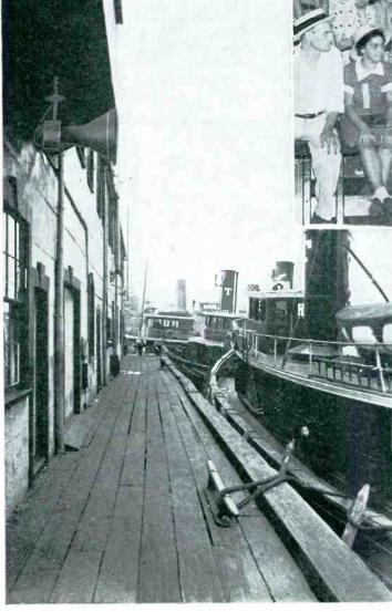
TUGBOAT TALKBACK — Inter-communicating system on a large scale is the installation on the docks of the Boston Towboat Company. A mike installed in the office by Eastern Radio permits officials to talk to captains, who answer back from their own decks, the speaker working in reverse as the pickup device
