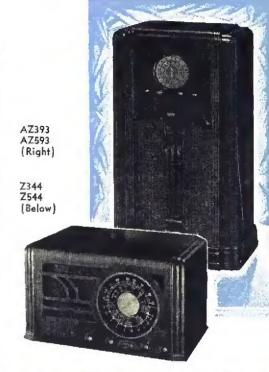
Model Z344 Admiral 6 tube AC "Laydown"—3 fubands. 6\%" airplane dial, 3 watts undistorted outpu "Hi-gain" colls for better selectivity and sensitivity 3 gang condenser. Plug-in type heavy duty dynami speaker, Antomatic volume control. List price \$39.98
