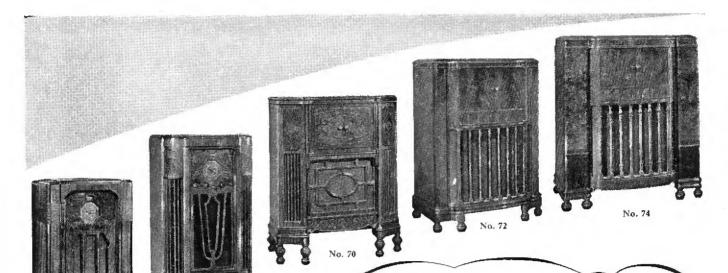
THE NO. 58 SERIES. Triple Range, glass tube radios with the "Cloverleaf" wiring of coils and range switch.
