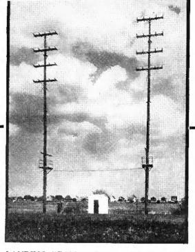
LANDING BEAM equipment installed by the Department of Commerce at Newark Airport for experimental use permits a plane pilot flying blind under a cockpit hood to set his wheels down without a crash simply by watching instrument panel indicators. Picture shows part of the antenna system which emits both a directive and landing beam
