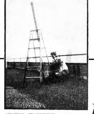
AMATEUR TRANSCEIVER made by Gross Radio operated atop the McGraw-Hill Building in New York contacts Manhattan and New Jersey "hams" on 5-meters. Many units of this type are already being marketed by radio dealers. (Empire State Tower, from which experimental television signals are transmitted on 7-meters, in background) Radio dealers will eventually feel the effect of these newly developed services, furnishing replacement tubes and parts, if not original equipment
