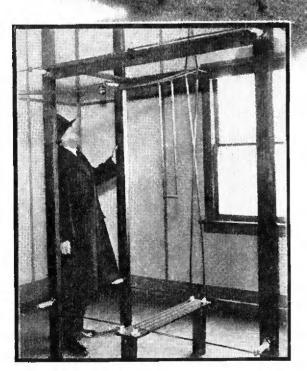
TELEPHONE SERVICE between Provincetown, Massachusetts, and several points on the "Cape" difficult to reach by land-line is maintained by the Bell System through a radiophone link. Here are the directional ultra-high frequency receiving and transmitting antenna arrays. The equipment is not attended, works automatically
