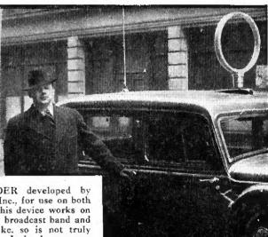
DIRECTION FINDER developed by Lear Developments, Inc., for use on both a reraft and ships. This device works on signals in the regular broadcast band and from 3,000 to 6,200 kc. so is not truly ultra-high frequency. It is, however, a new development in shortwave equipment
