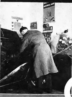
BOUNCING THE SET five inches onto the wooden bench-top while it is playing, prior to installation, shows up loose parts and faulty joints. Rough, but no more so than the road
