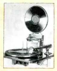
Model 10-12 in loading position. Note the lever on right side which throws the unit into position for 10-inch records when down or 12-inch records when up. With a special arrangement incorporating a double-throw master switch, one record can be placed on the turn-table, the adjustment set according to the size of the record and the magazine can be loaded while the pick-up automatically comes into position and the first record is being played.
