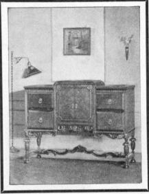
Model 255, a magnificent combination radio (six tube, single dial, Loftin-White circuit) and electric phonograph, operating directly from the lamp socket.
