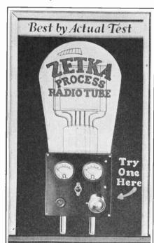
The above counter display stands 22 inches high and contains a tube tester made up of Weston instruments mounted on a small bakelite panel. A rheostat located in one corner controls the filament voltage, and the push button in the center operates a safety circuit, so that in case the tube elements are short-circuited no damage will be done to the meters.
