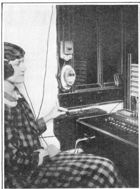
By a System of Relays, the Telephone Operator at Her Switchboard on the Ground Floor is Able to Control the Robert Morris Hotel Radio Receiver, Located on the Fourteenth Floor. The Installation was Designed to Give Earphone Volume in 208 Rooms.
