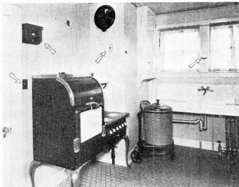
Sink light, outlet for ventilating fan, annunciator, wall switch, dishwasher, and range are some of the electrical service features in the kitchen of the Detroit home electrical. Adequate wiring did it. A demonstration is helpful in selling the wiring idea.
