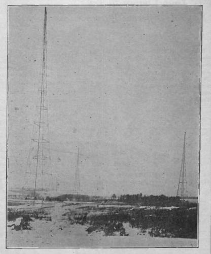
Fig. 3. Three Steel Masts Tower Above the Laboratory Lot. They are 300 Feet High
