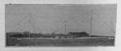
Fig. 4. Wooden Masts Must be Used for the High Speed Waves, as Shown Here
