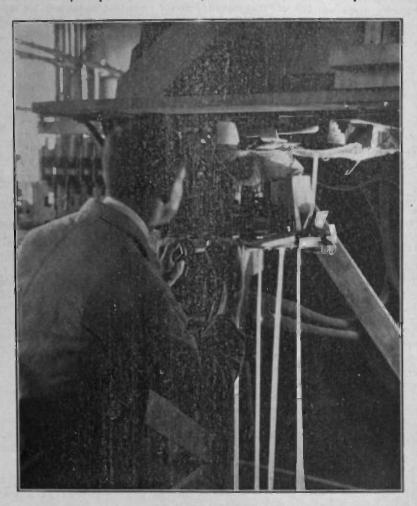
Fig. 4. Details of White-Hot Tubes Flowing from Furnace. Notice Heavy Leads Which Carry the Electric Current
