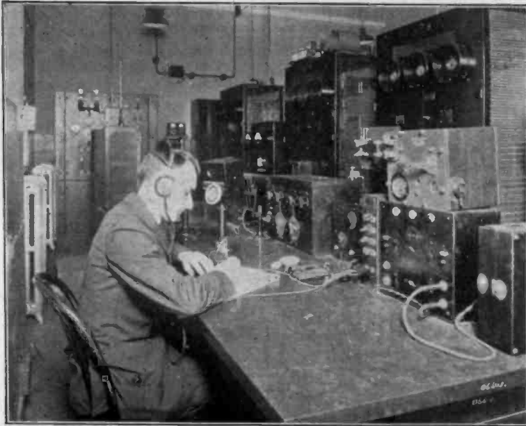
Fig. 2. Relays and Switches for Re-Broadcasting
