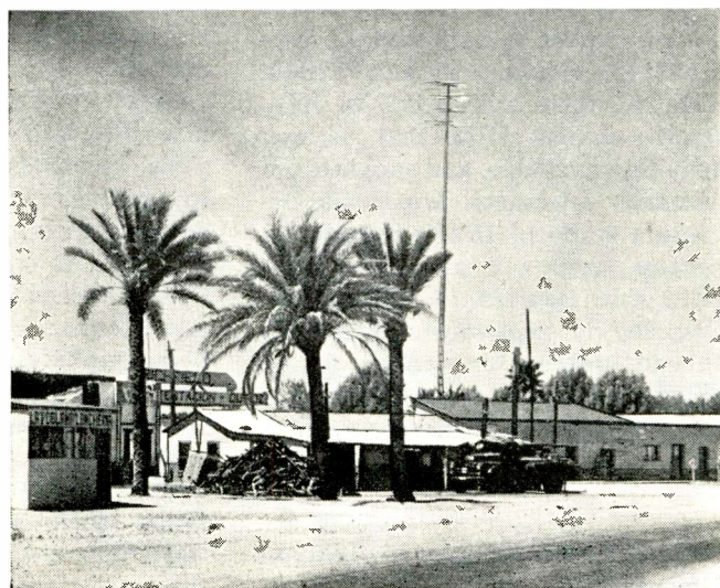
Fig. 3. An antenna installation at Sonoita, Sonora, Mexico. Rather good reception is the rule here although the nearest TV stations are about 200 miles away and all power is generated locally by a diesel plant of small size.
