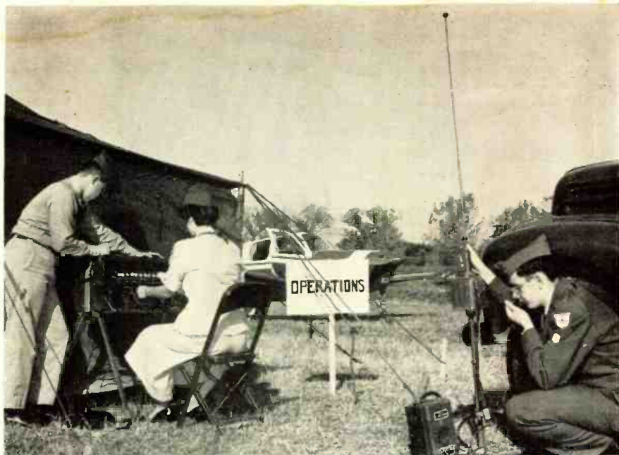
A Cadet operates an SCR-511 "Pogo Stick" high-frequency transceiver, relaying instruction to CAP aircraft engaged in disaster relief training mission. Cadets at left operate a telephone switchboard tied into the local Civil Defense agency.
