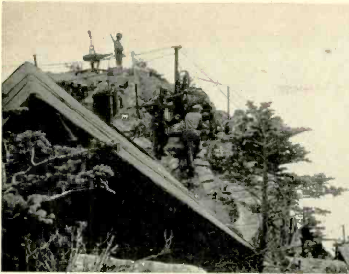
View of one of the cloud-topping relay stations. Korean guards, operating personnel, and antennas are visible among the boulders.
