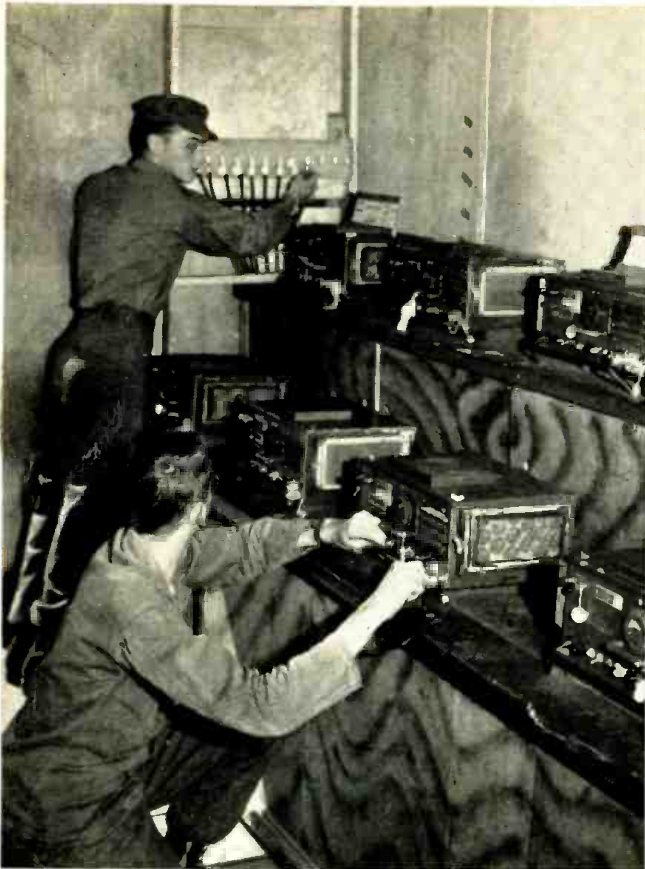
Pfc. Lawrence R. Jackson and Sgt. Gorver W. Potter, radio-men, switch receiving antennas at a v.h.f. relay station site.
