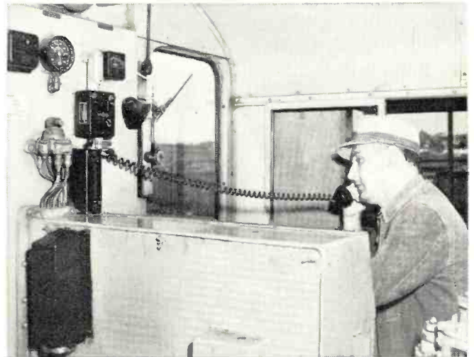
Engineer on a diesel switch engine keeps in touch by radio.
