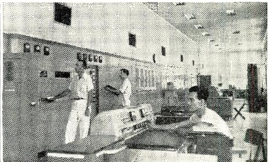
Transmitters of the "Voice of America" relay station at Manila, Philippines.
