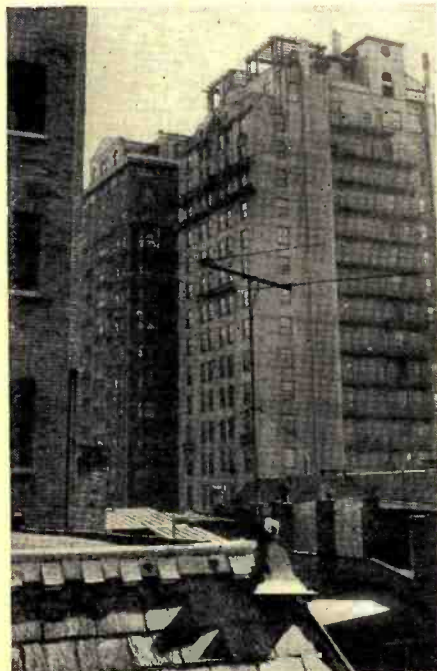
Fig. 6. Photograph shows a typical urban installation where a conventional dipole and reflector antenna is used to provide adequate reception on the two preferred TV channels as selected by the customer.
