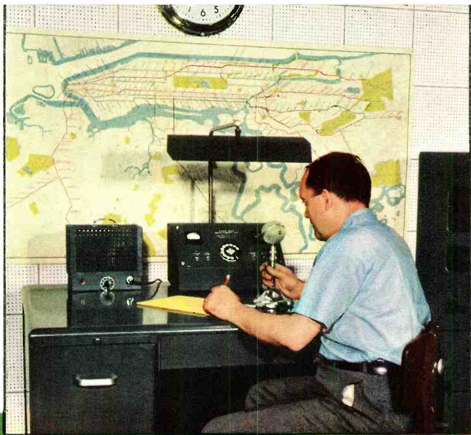
Control office of Queens Midtown Tunnel experimental installation may be used to transmit programs, emergency warnings, and traffic instructions to tunnel users instantly. All repeated instructions are sent by magnetic-tape recorders.
