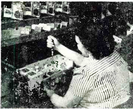
Mounting trimmer condenser on transmitter chassis. Junction blocks are on rack.
