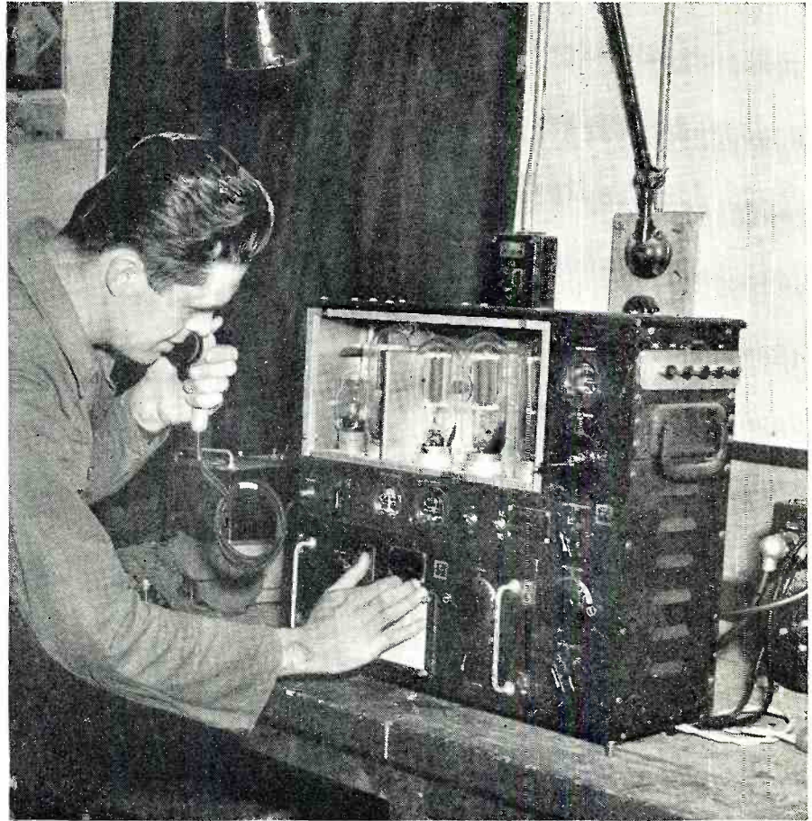
Completing the final testing of a repaired transmitter which will again be used. This transmitter is one of seven complete radio-sets installed in all Flying Forts.
