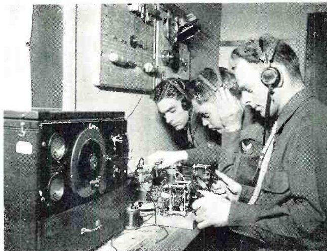
Part of Basic Receiver Laboratory where students build and operate breadboard-style receivers. Every part of the chassis is exposed for study.
