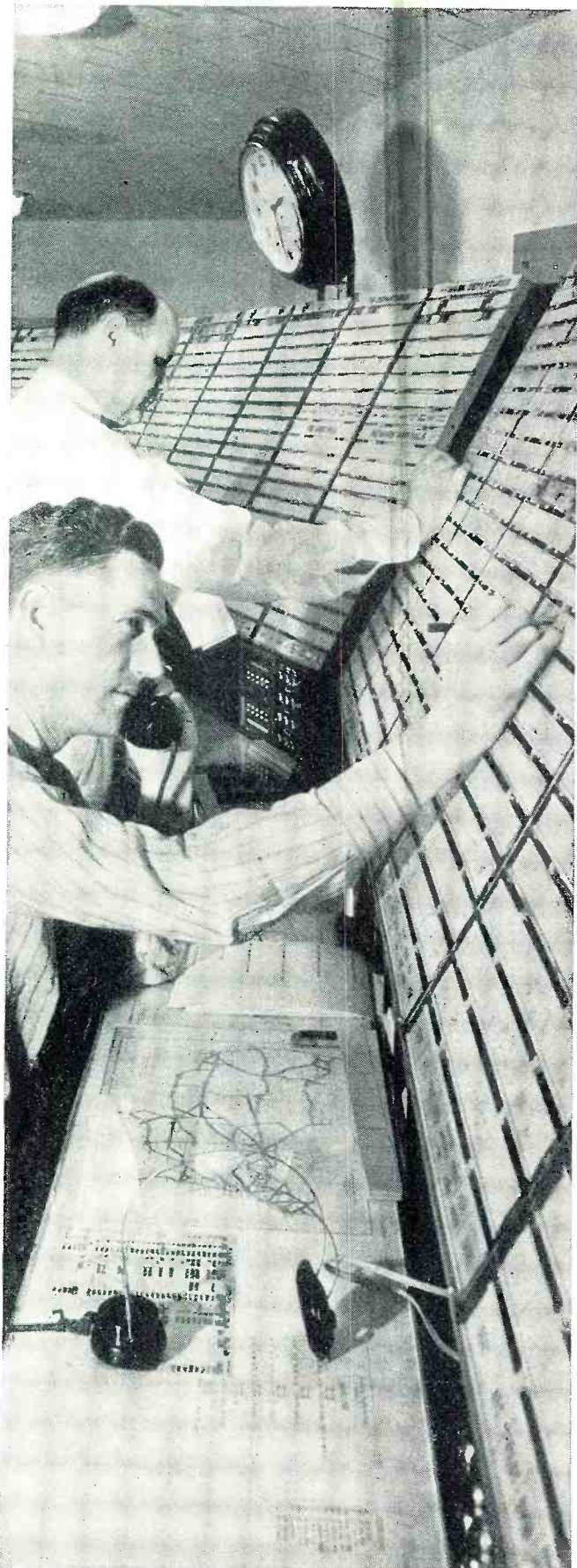
Typical Airway Traffic Control Center equipped with manually operated Flight Progress Boards. An elaborate communications system, both telephone and radio, is necessary to record position of all planes in flight.
