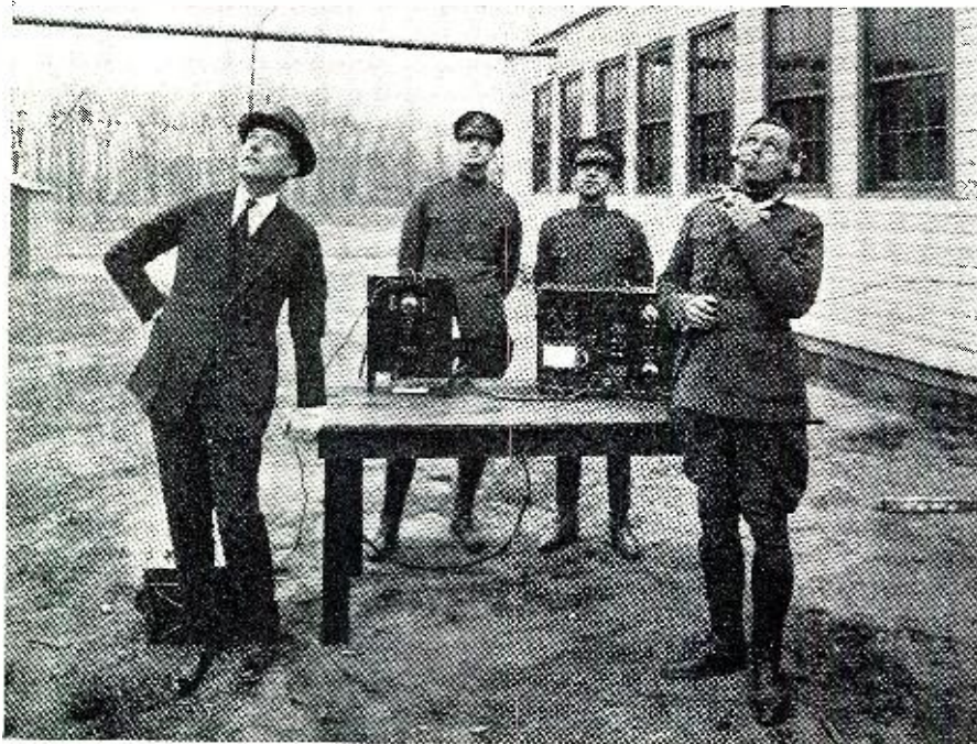
Experimental aircraft radio telephone installation during World War I (1917).
