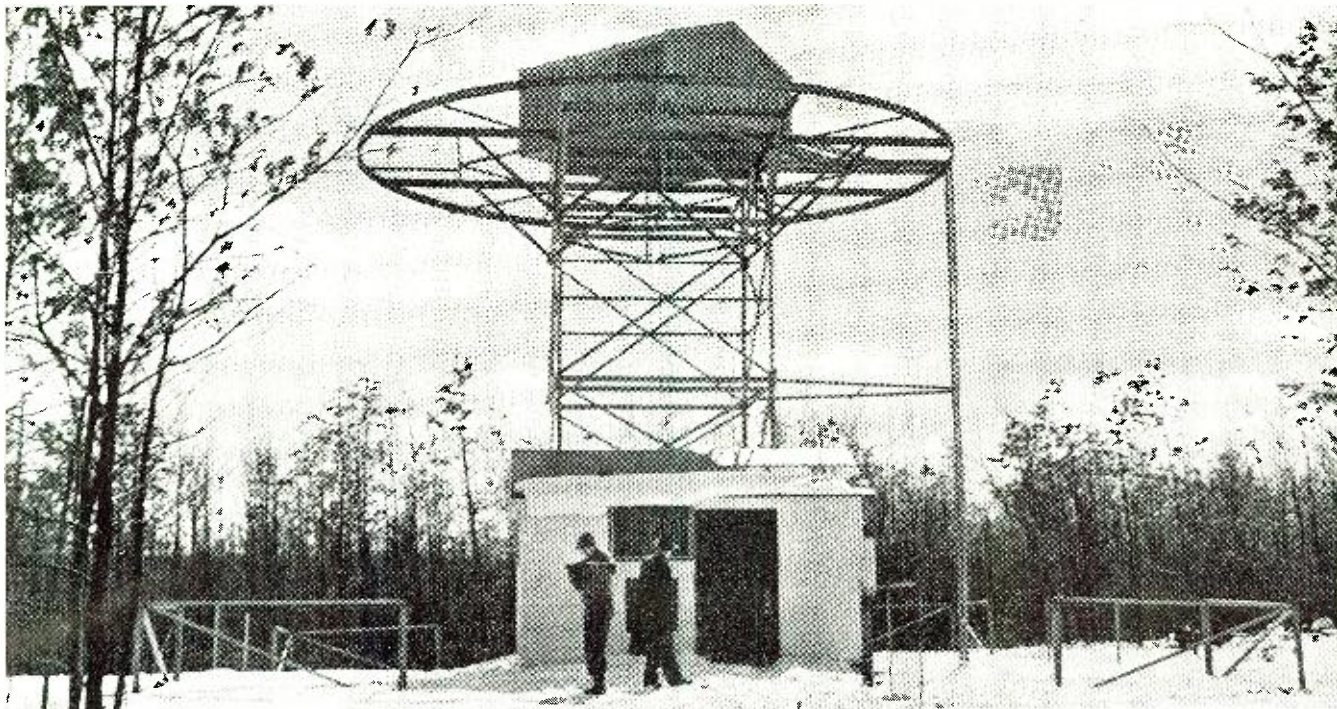
Ultra-high-frequency four course radio range station, needed to safely operate our many airways.
