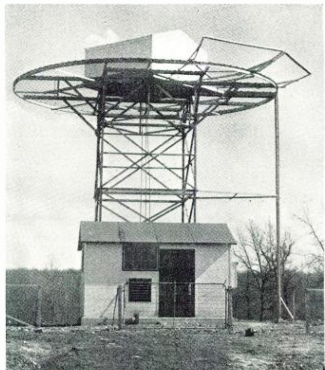
Fig. 2. Tower and building for UHF ranges. Many similar units will be needed to provide complete airway coverage.
