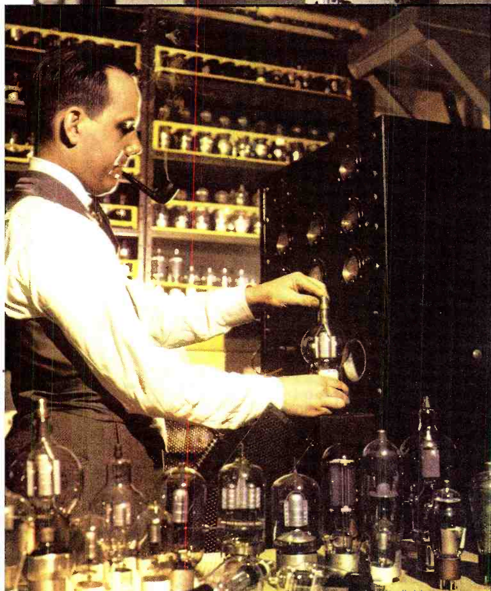
Specially-designed 20kw. transmitters at the CAA intercontinental radio station, Sayville, L. I., have world-wide coverage. Air-cooled tubes are used.
