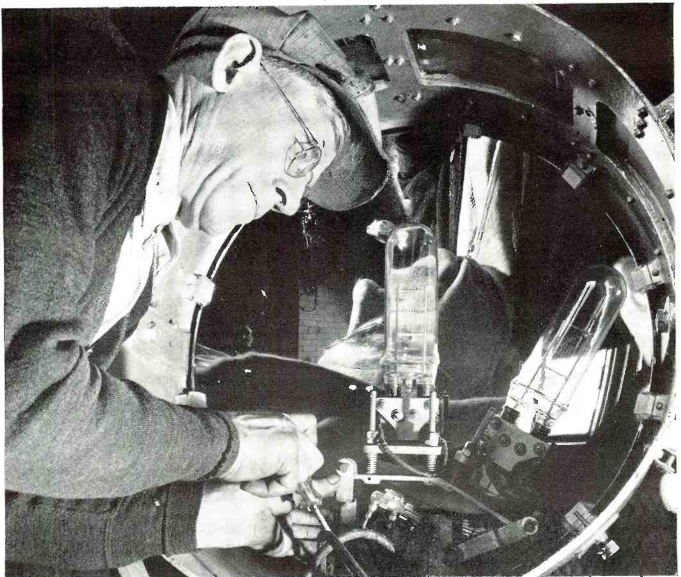
Maintenance check on airways beacon light. This one has a 36" diameter lens.
