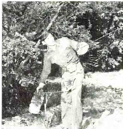
Stretching antenna to nearby tree. Second wire gives directional effect.
