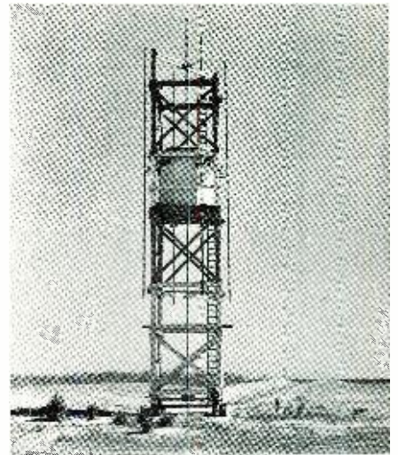
Antenna system for azimuth indicator beam.
