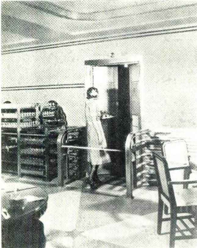
These kitchen-to-dining room doors open automatically.
