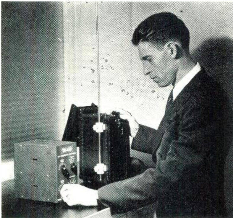
Checking frequency of the portable against crystal-controlled standard.
