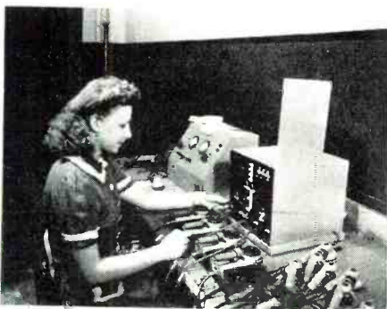
Operator checks microphones to see that they are in perfect condition.
