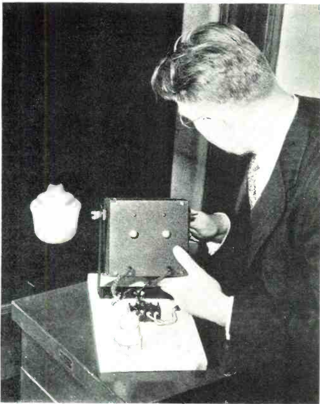
G.E. blackout photoelectric eye focused on streetlight.
