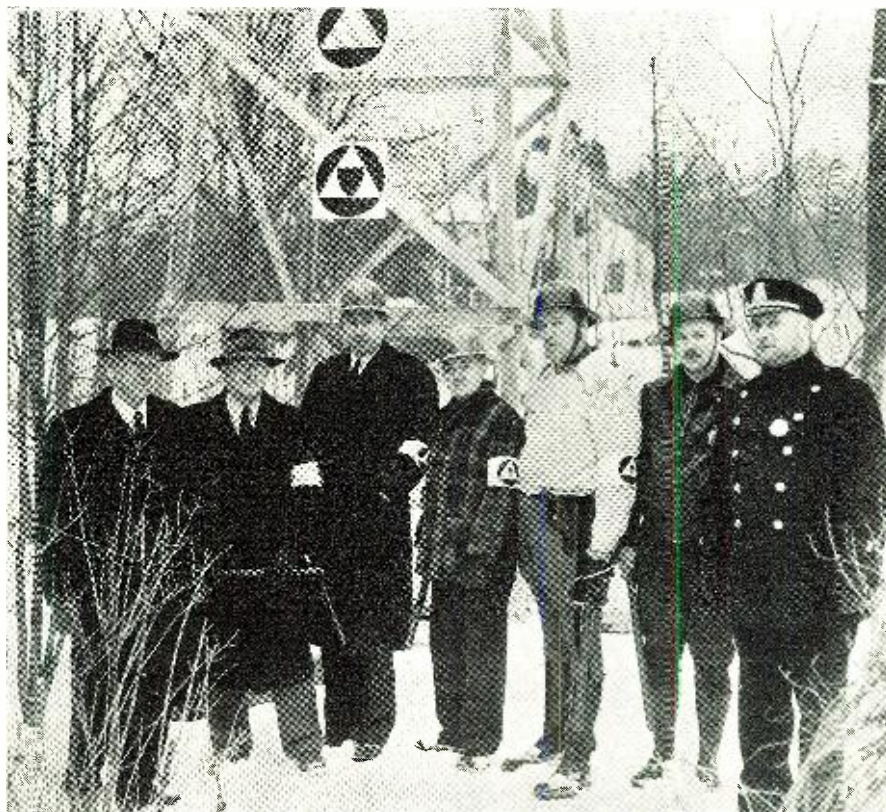
These A.P.'s cooperated in constructing this project and operate the system.
