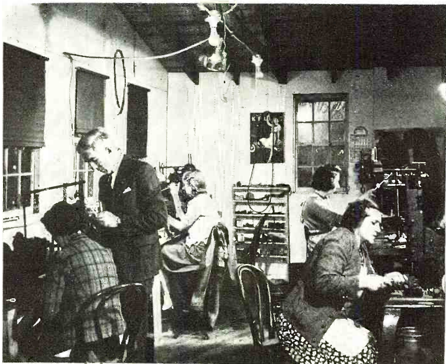
Women workers of electric company inserting screws into terminals.
