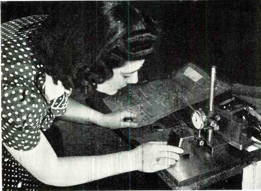
Razor plants turn out precision parts. Operator checking V block.
