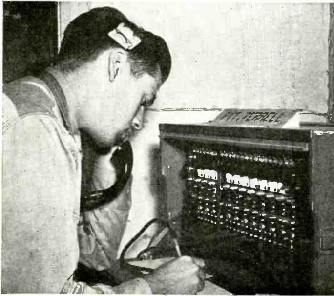
This portable telephone switchboard may be transported into the field and placed in operation in quick time.
