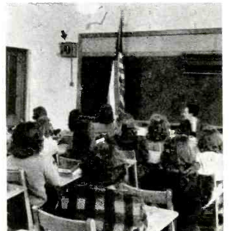
Wall-type speakers installed by students in one of the classrooms.
