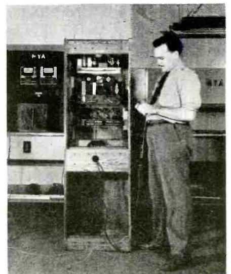
Every joint is carefully checked to assure the best performance.
