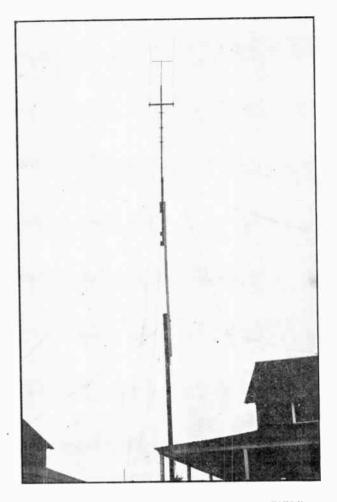
THE DOUBLE "J" INSTALLED AT FAIRFIELD This highly efficient beam antenna, atop a 60-foot collapsible mast, has been doing fine work at W2JCR's portable location in Connecticut.
