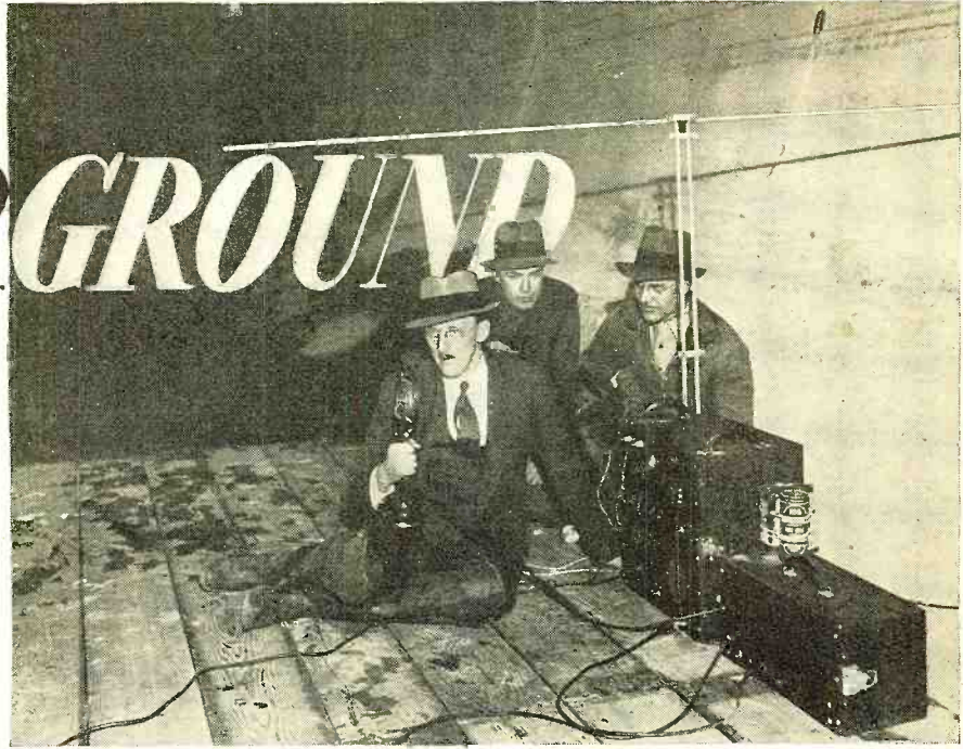
SEMI-PORTABLE RIG MOUNTED ON TUNNEL PLATFORM
