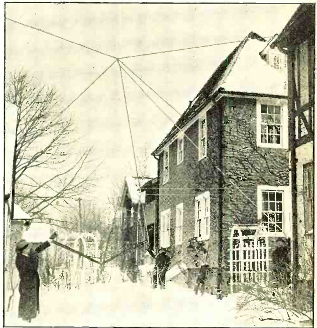
AERIAL INSTALLATION UNDER DIFFICULTIES
