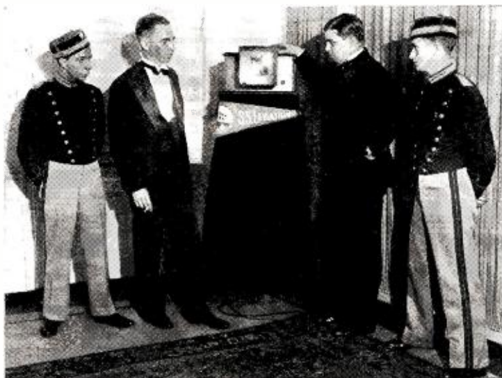
THE RADIOVISOR INSTALLATION ON THE LEVIATHAN
