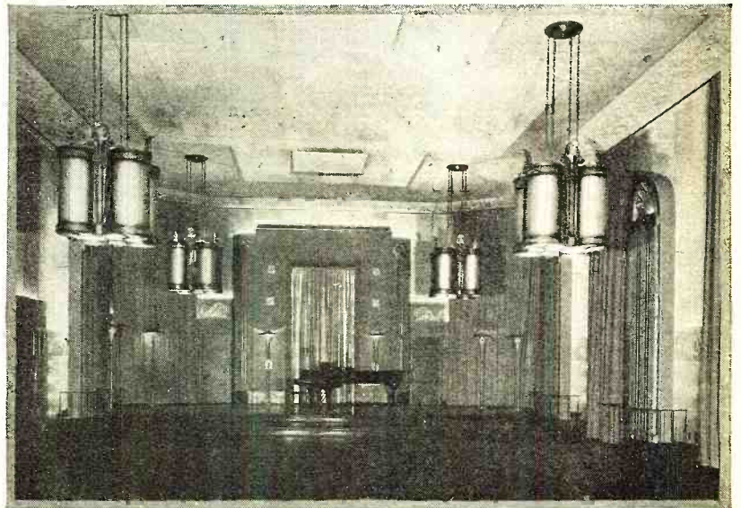
While the illustration above does not depict the interior of a theatre, it does illustrate how one of the larger of the NBC studios has been treated with sound-absorbing curtains, drapes, etc., so as to make for better quality of transmission without reverberation or reflection of sounds within the studio
