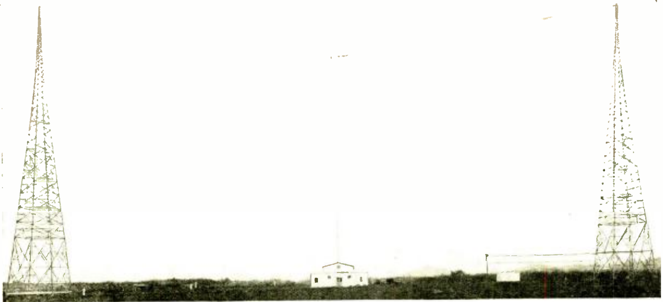
The towers of Station KNX after insulators have been installed in order to minimize their absorption effects
