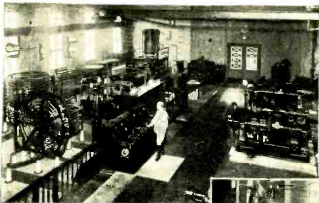
Above, the generators and transmitting equipment of broadcasting station at Königswunsterhausen, Germany, from which programs were transmitted on short waves to the United States on Christmas Day. Right, control room of the Königswunsterhausen station
