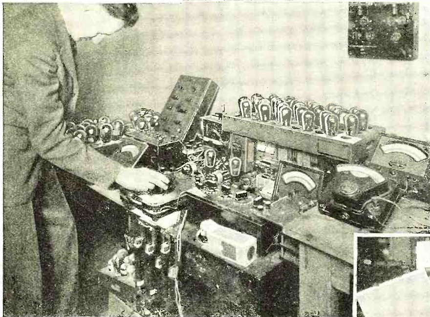
¶ Fig. 12—Completed tubes are allowed to “age” for a length of time, which varies according to the manufacturer’s own schedule
