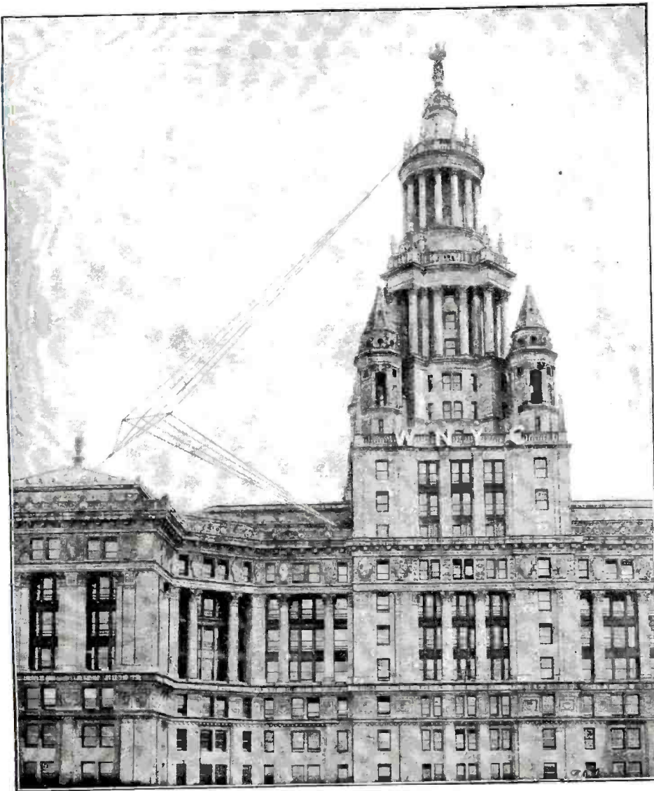
The transmitting aerial of WNYC, atop the 40-story Municipal Building, which looks down on New York's historic City Hall. The aerial has recently been rearranged, as shown here.
