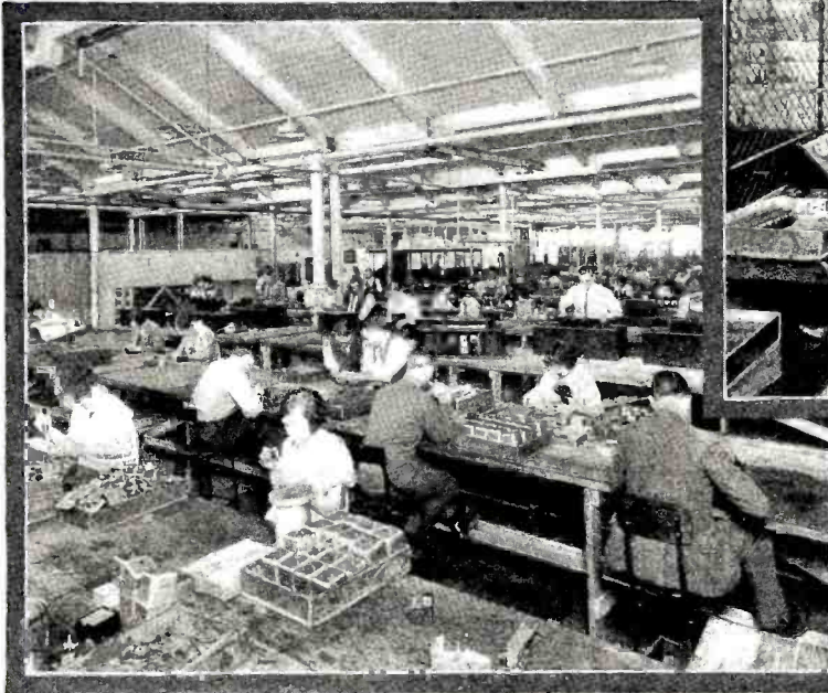
↑ Above we see a big assembly room, where the units of parts from the various stamping, winding, and other machines are brought together, and united into complete apparatus by deft operators. Long stretches of benches can be seen in well-lighted rooms, where one operation follows another in quick succession. The suitable routing of assembly work is one of the greatest factors in high-quality and low-cost manufacture today.
