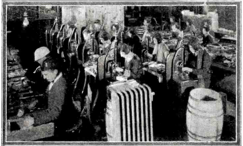
The capacity of the up-to-date condenser is determined before the final assembly, shown above, so that errors may be easily rectified.
