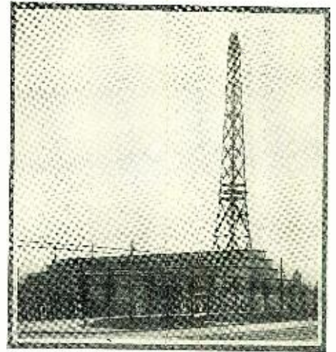
The exhibition hall built especially for radio in Berlin. The tower is the highest in Germany used for radio.
