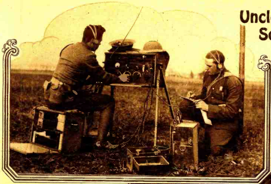
A PORTABLE FIELD SET. This signal corp sergeant saw service in France with the first division and knows a good shell hole when he sees one. It took him but two minutes to erect this battalion radio set; it was carried by two men, and establishes communication with a division set. This is all a part of the day's work at the Signal Corps School for the army at Camp Vail. (By United.)
