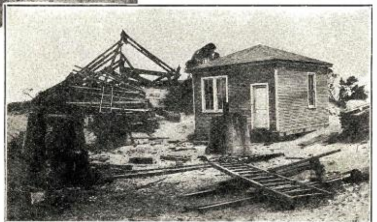
One of DeForest's first commercial stations and what happened to it in a high wind. The shack was built directly under the mast. H. P. Vosberg was chief operator.
