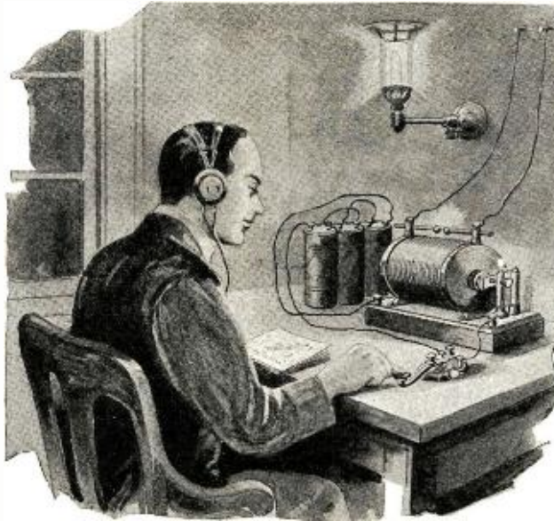
DeForest noted the change in brilliancy in a Welsback gas burner when his spark coil was in operation giving him the idea for the Audion.
